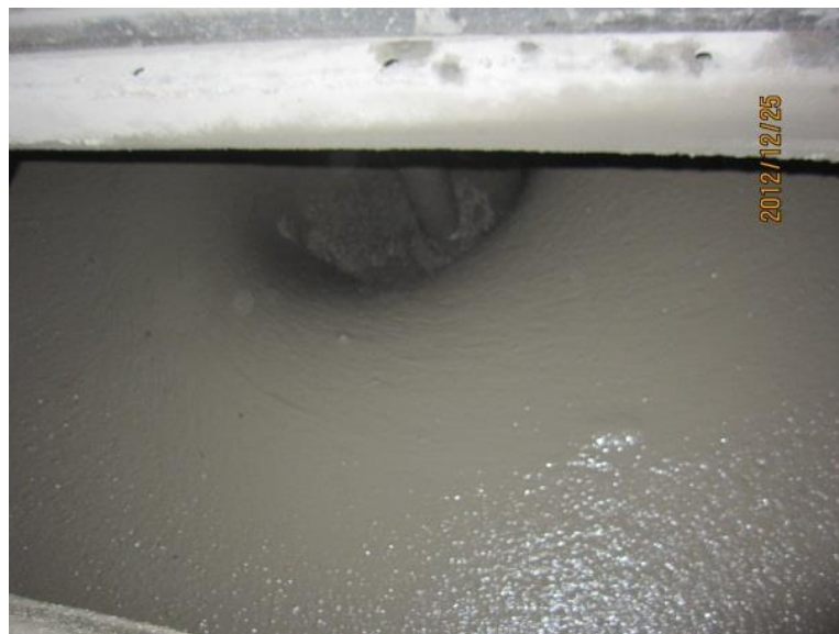
Figure 1 Mixing high-density slurry composed of sand (-3 mm), cement and water
