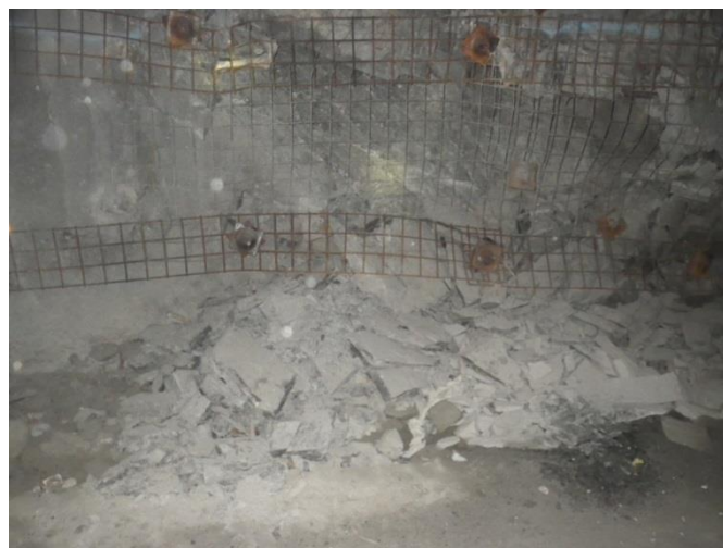
Figure 13 Small damage (R1) following seismic event M_{\text{Richter}} 2.0
