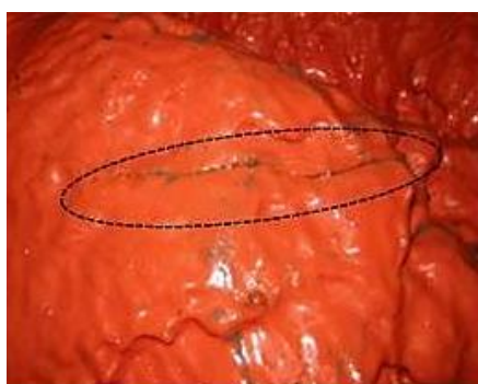
Figure 5 Small crack in full composite consisting of primer and 4 mm top coat (Boeg- Jensen 2013)
