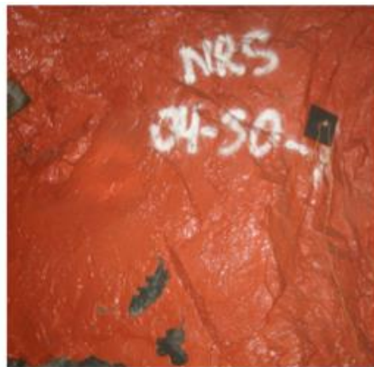
Figure 7 Scoop damage on the lower part of the wall for 8 mm top coat (Boeg-Jensen 2013)
