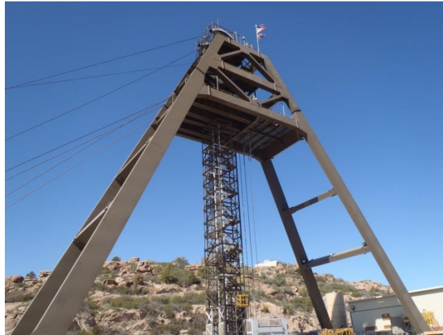
Figure 1 Resolution No. 10 Shaft Headframe, located near Superior, Arizona, USA
