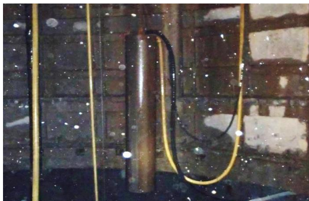
Figure 6 The hanging sump in operation
