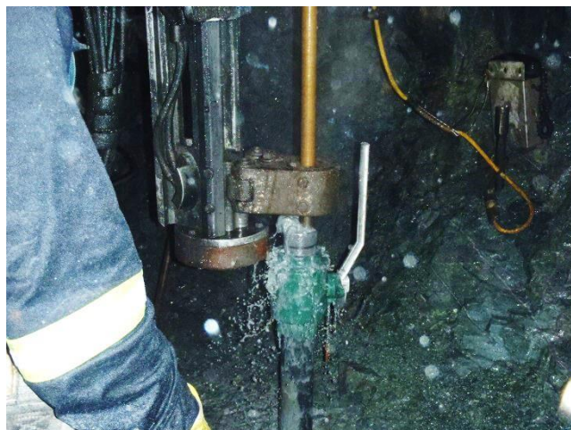
Figure 2 A cementation miner using a pneumatic jumbo rock drill to drill a 25 m probe hole on the 1,969 m bench
