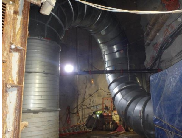
Figure 12 Exhaust line tie-in to the exhaust duct mid-shaft
