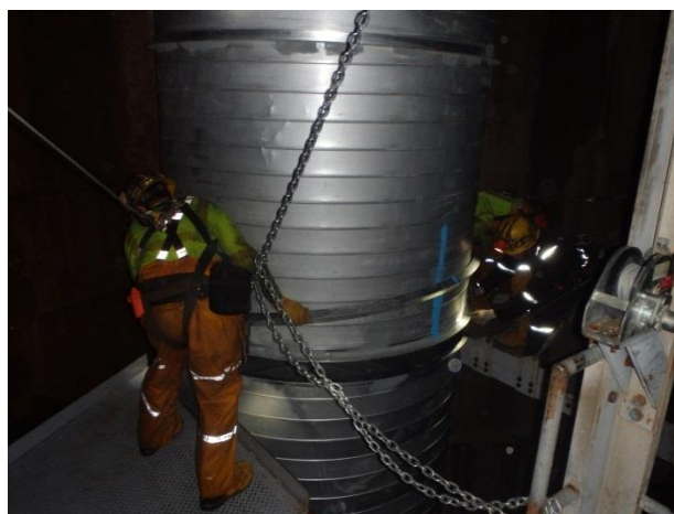
Figure 11 Installation of the 2 m diameter exhaust fans at the Pump Level
