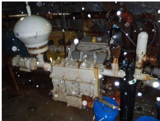
Figure 9 One of two positive displacement pumps installed at the Set 326 Pump Station
