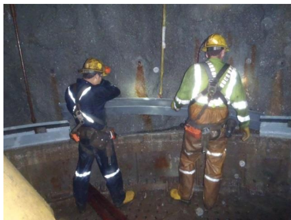
Figure 5 The installation of a water ring during a shaft liner pour
