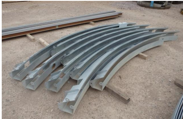
Figure 4 Sections of a water ring on surface before installation
