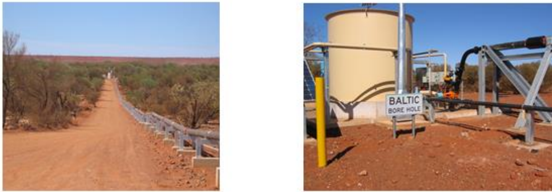
Figure 3 Delivery line to site of placement of backfill material
