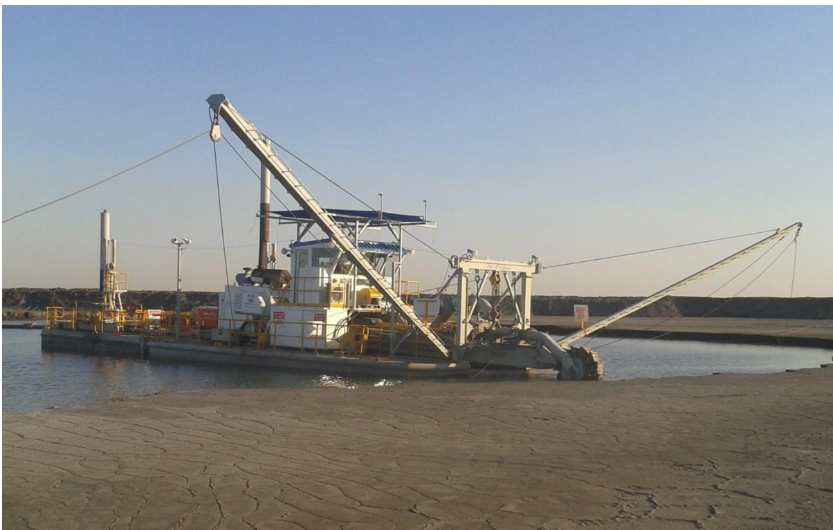
Figure 4 A photograph of the dredge at work. The bucket-wheel cutter has been raised above the pond surface, and can be seen at the front of the dredge
