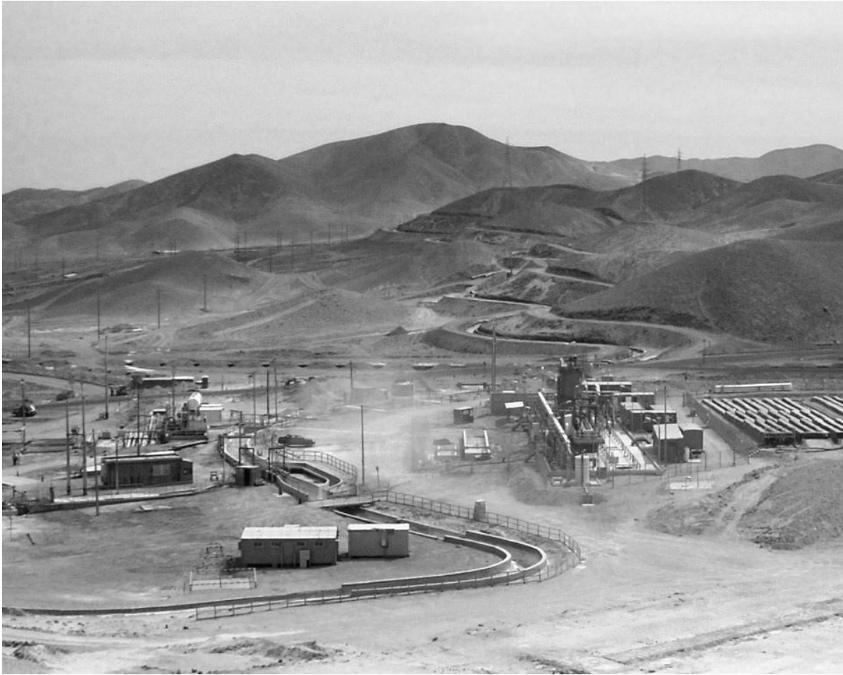
Figure 1 The tailings launder at the Chuquicamata copper mine, Chile
