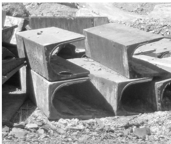
Figure 3 Precast U-shaped sections from a tailings launder at a mine in Australia
