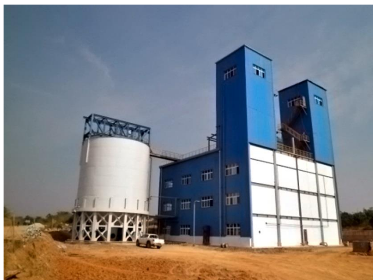
Figure 1 Overview of the paste plant at Chambishi
