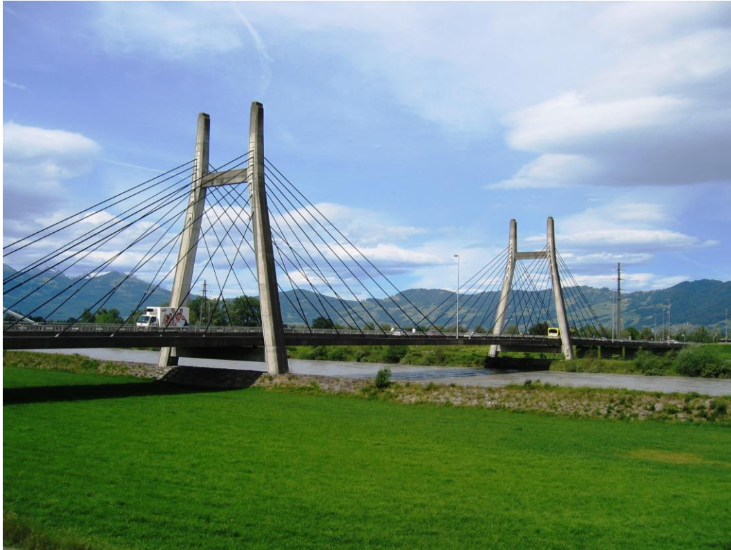
Figure 1 The Rhine Bridge — the object of monitoring
