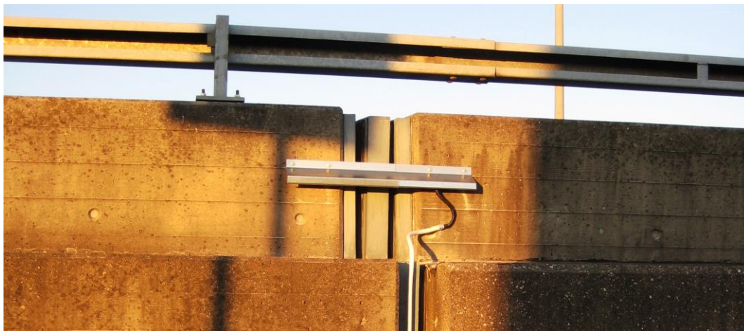
Figure 5 Mounting of the extensometer at position 1
