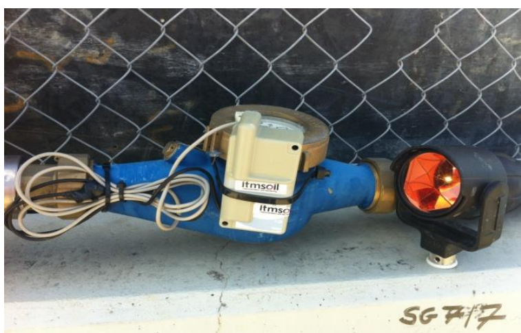
Figure 3 Rippa connected to water meter
