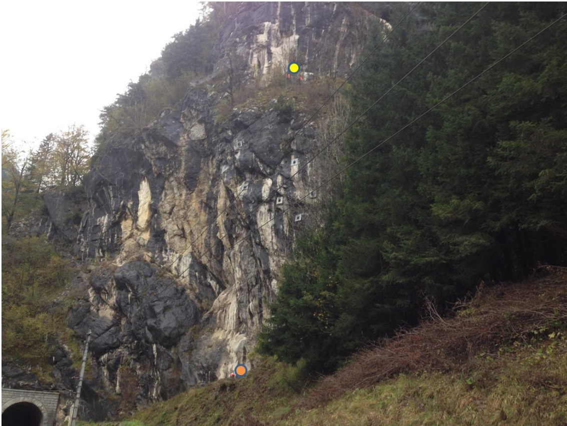
Figure 6 Hieflau tunnel, central Austria
