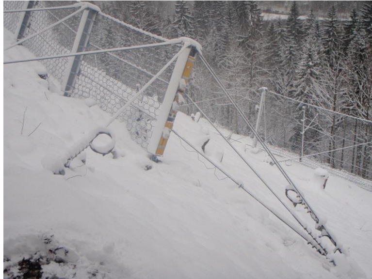
Figure 7 Rockfall barrier, central Austria
