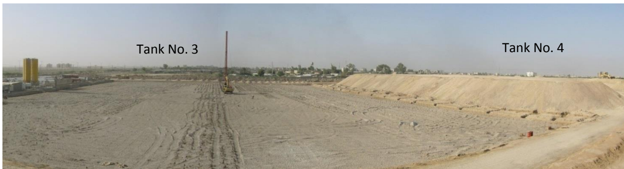
Figure 2 Position of two water tanks
