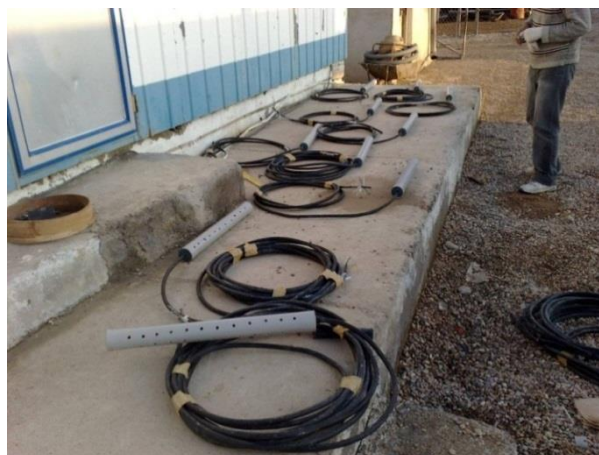
Figure 3 Protective PVC tubes for vibrating wire piezometers
