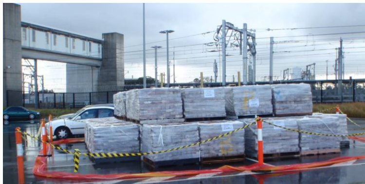
Figure 3 Example of large-scale in situ load test using brick pallets and precise surveying
