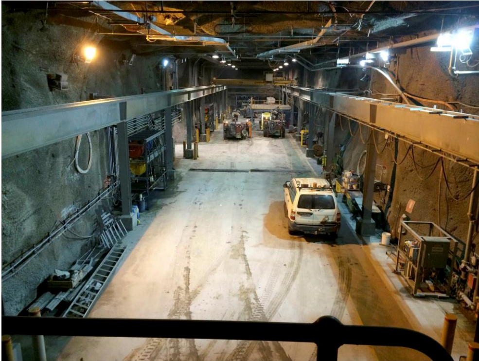
Figure 6 Extraction level workshop
