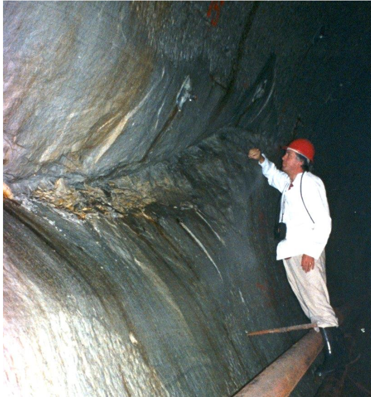
Figure 11 Stress-induced breakout in a bored tunnel at a depth of 150 m
