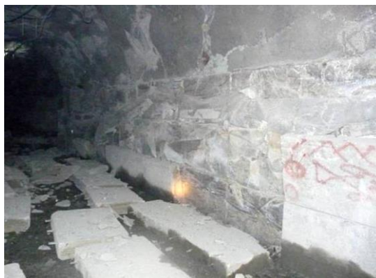
Figure 16 Concrete support panels ejected during a rockburst event (Stacey & Rojas 2013)
