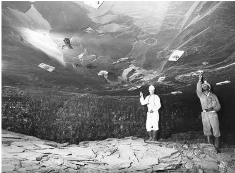
Figure 6 General view of the roof failure
