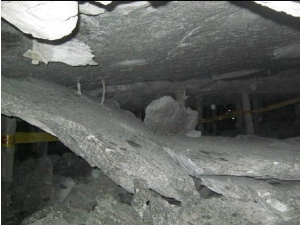
Figure 9 Dynamic roof failure in a tabular platinum mine stope (Stacey & van Rooyen 2014)
