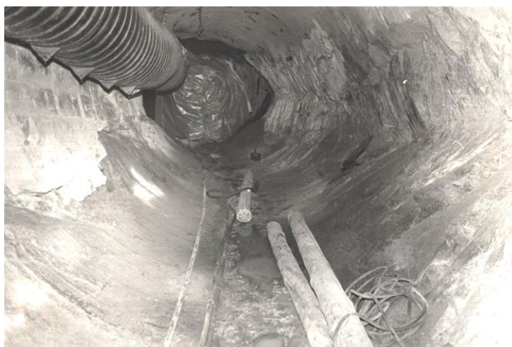
Figure 10 Bored tunnel in a high stress gold mining environment
