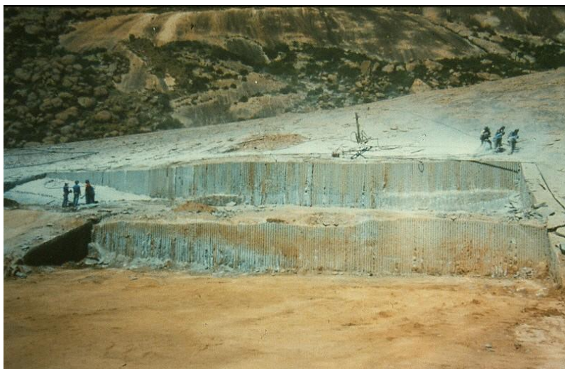
Figure 4 Extent of the quarry
