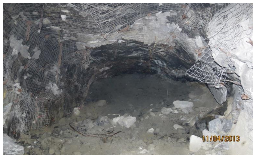
Figure 2 9410-140-27, stope overcut showing stress arching (looking towards hanging wall contact)
