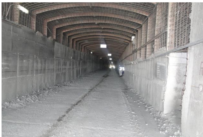
Figure 3 South ramp (5.5 × 5.0 m)
