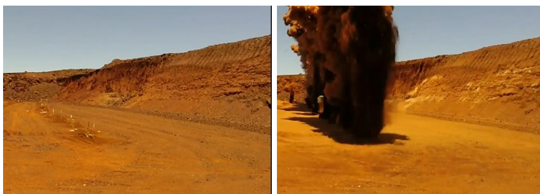
Figure 6 Absence of dilation in bench behind un-stemmed buffer blastholes (12 m bench, 251 mm diameter)
