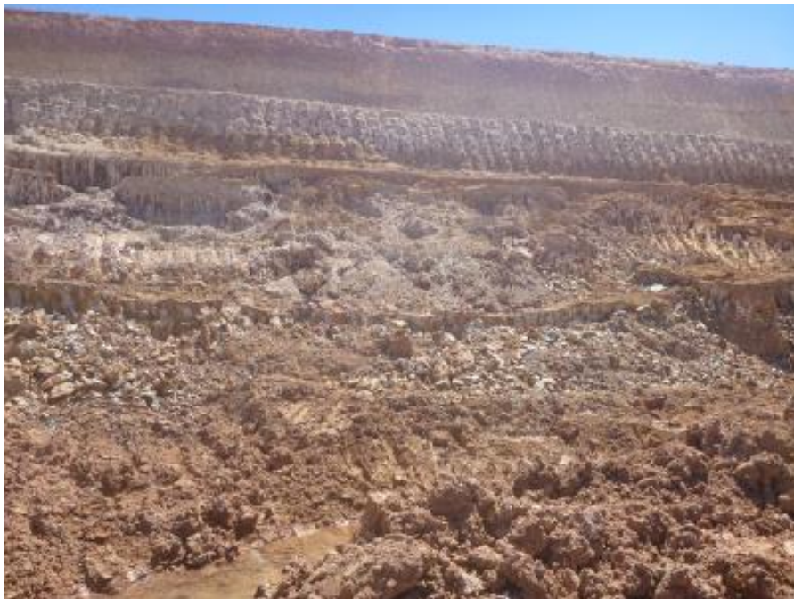
Figure 12 Photograph of slope failure
