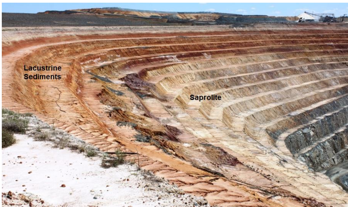
Figure 13 Multi-bench failure at the base of the lacustrine sediments
