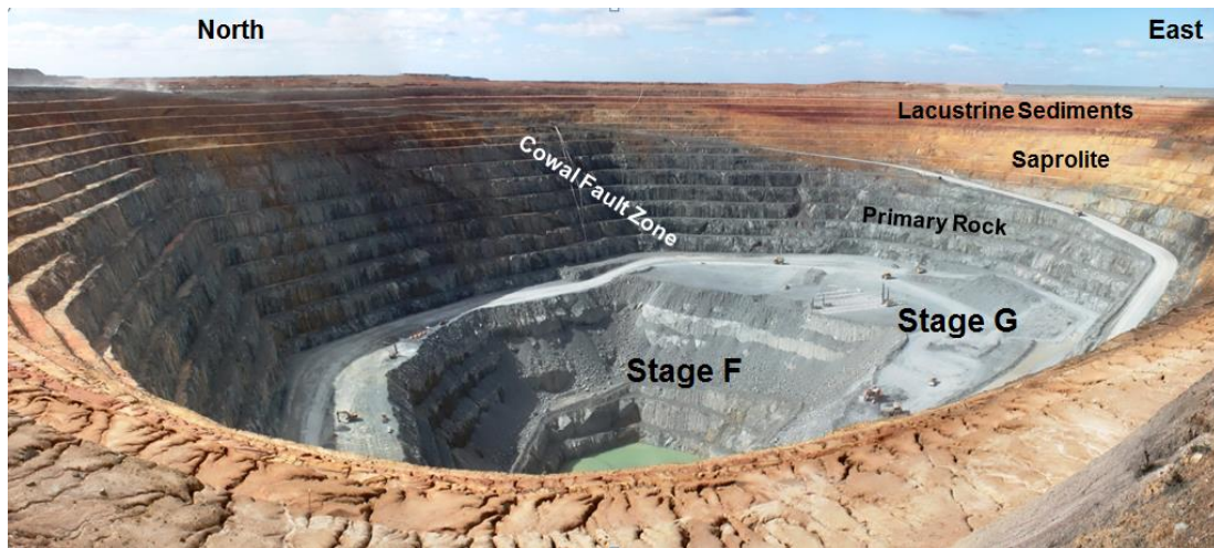
Figure 14 Pit as of 15 March 2015
