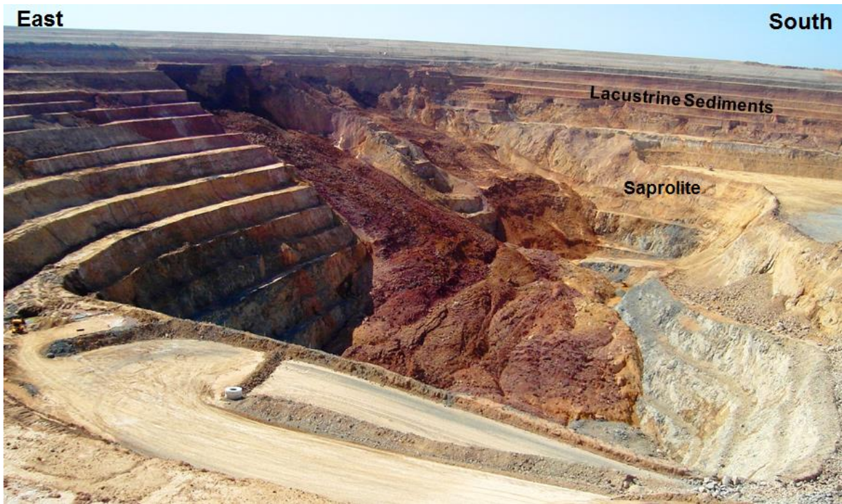
Figure 2 East wall failures — December 2007
