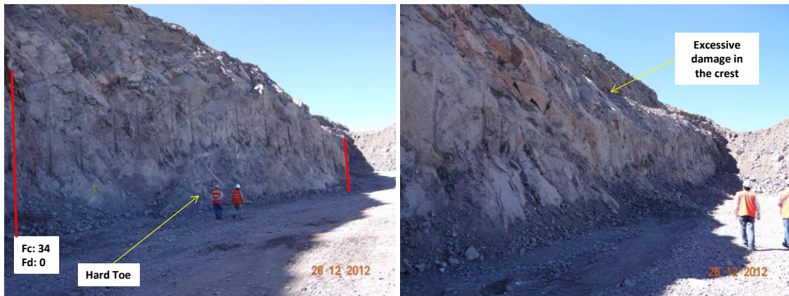
Figure 10 Results of contour blasting test 1
