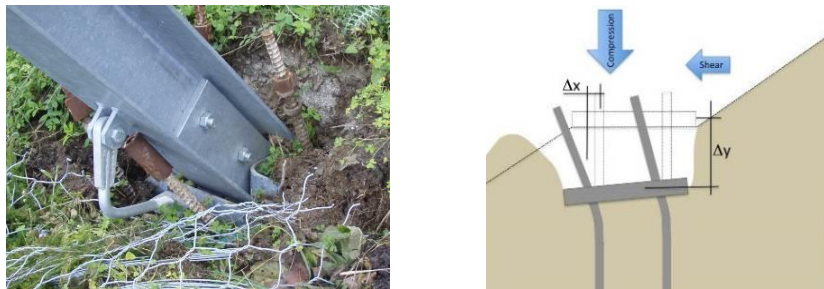
Figure 11 Settlement of the footplate after the impact. The vertical ( \Delta y = approximately 200 mm) and the horizontal ( \Delta x = approximately 50 to 100 mm) displacements of the base plate represent a benefit for the energy dissipation of the fence
