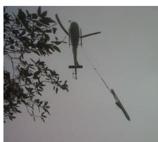
Figure 9 Installation of the barrier post using helicopters
