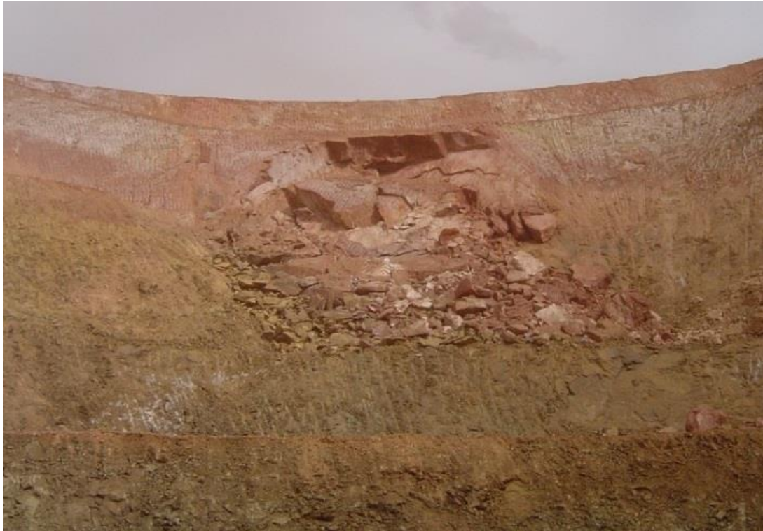
Figure 1 View of the failure from below
