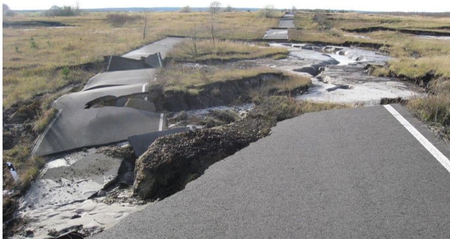
Figure 7 Ground-break at a street at the former Schlabendorf-South mine in 2015 (source: LMBV)
