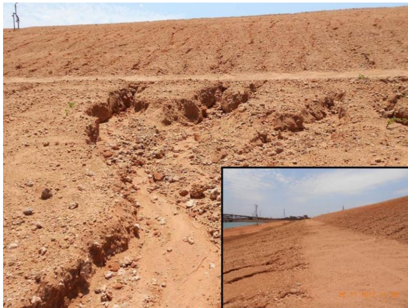
Figure 15 Waste landform rilled upper batter, and gullied lower berm, and filled forward sloping berm (inset)
