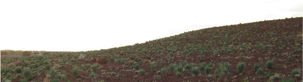
Figure 18 Concave slope profile (designed based on measurements of erodibility) used to stabilise a waste dump batter in the Goldfields (no berm required)
