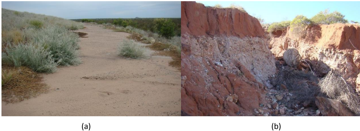
Figure 3 (a) Back sloping berms filling with sediment; (b) ponded dump top runoff overtopping and discharging to batter slopes
