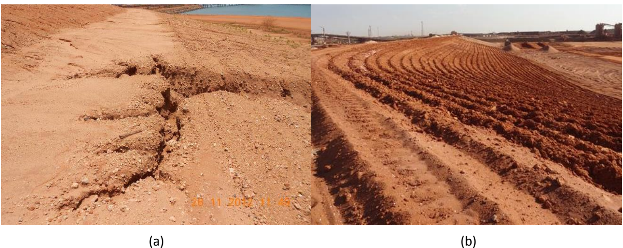
Figure 9 (a) Rehabilitation of a marine dredge spoil bund showing failed berm; (b) reshaping to remove berm and add rock into the surface
