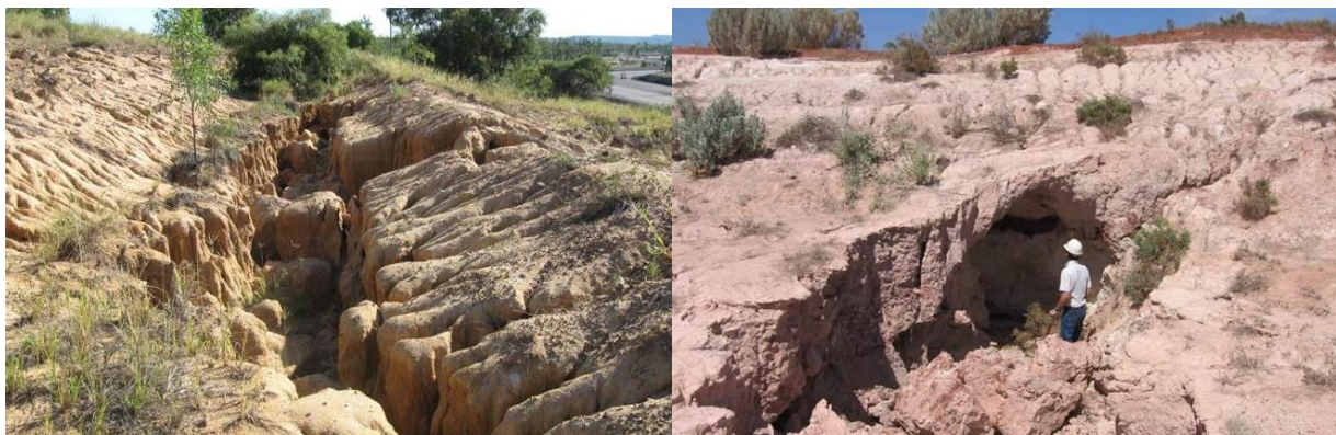
Figure 4 Tunnel failure on berms constructed with tunnel-prone material
