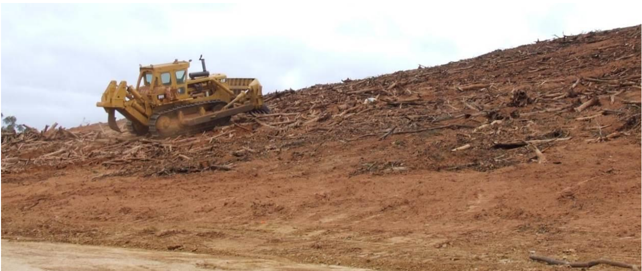
Figure 17 Addition of tree debris to increase erosion resistance of a batter slope (eliminating berm)
