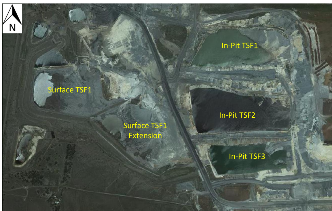
Figure 1 New Acland surface and in-pit TSFs (aerial photograph taken on 12 March 2013)
