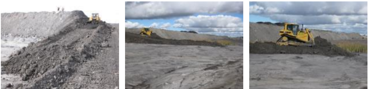
Figure 13 Early pushing of a capping of coarse reject over old bow-wave of surface TSF
