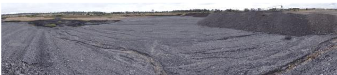
Figure 17 Progress of capping of surface TSF as at 25 June 2015, with all but the northwestern corner of TSF1 capped
