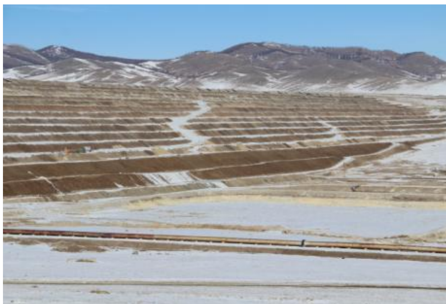
Figure 6 Upstream embankment design with valley and surrounding mountains at Erdenet Mine
