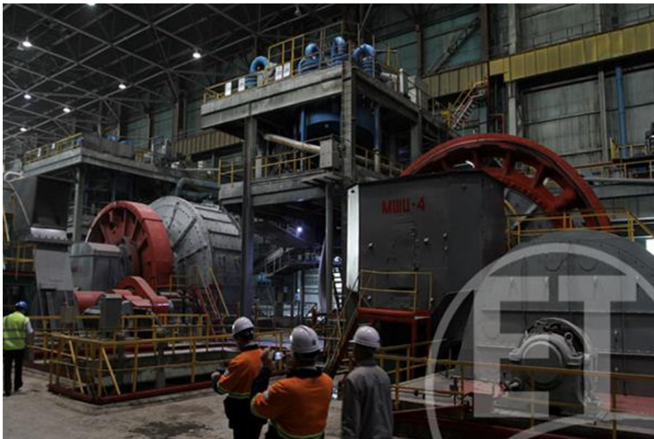
Figure 2 Erdenet Mine processing plant expansion
