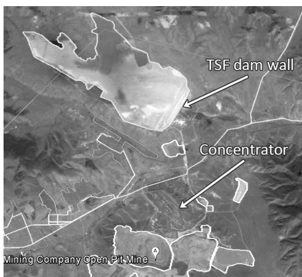
Figure 5 Erdenet Mine tailings storage facility overview
