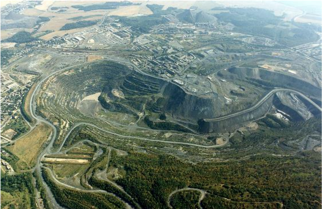
Figure 2 Lichtenberg open pit in 1990 (view from west to east)
