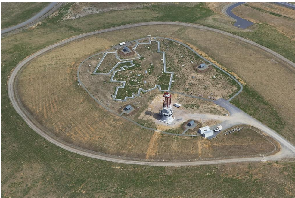
Figure 6 Top plateau of the hill Schmirchauer Höhe with park area (under construction)
