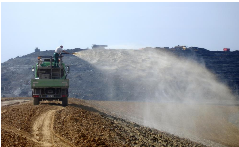
Figure 7 Hydroseeding on the subsurface of relocated dumps close to the open pit
