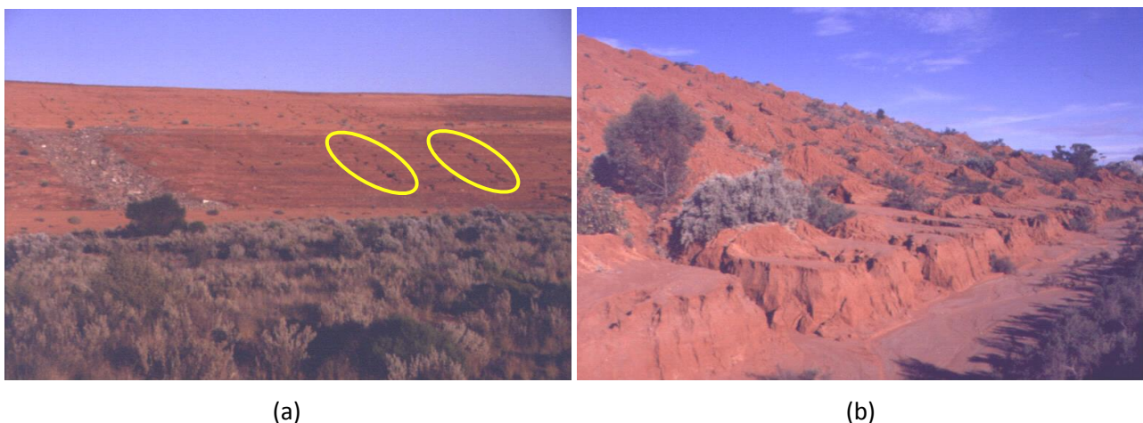
Figure 14 Waste rock dump flattened to 1 in 3, with contour and downslope drains constructed, and topsoiled, showing: (a) rilling away from downslope drain on first rainfall event, and (b) deep erosion gullies through thick topsoil over time
