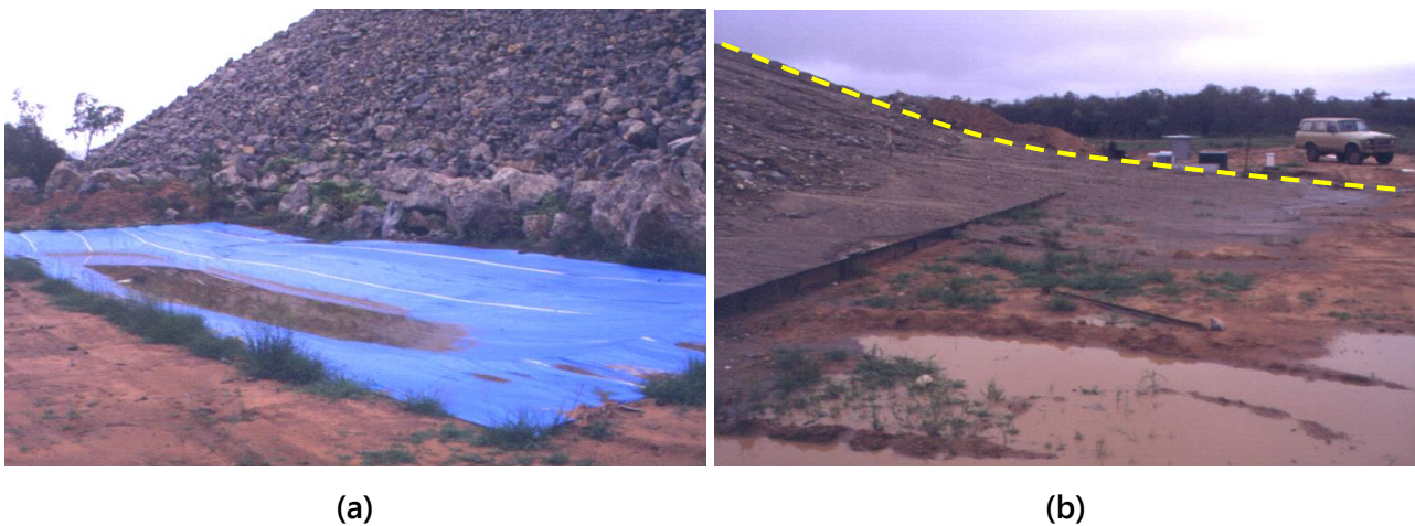
Figure 13 Waste rock dump erosion due to a 25 mm rainfall event, showing: (a) negligible erosion off an angle of repose slope, and (b) substantial erosion of a slope flattened to 1 in 3 and covered with a 500 mm thickness of growth medium
