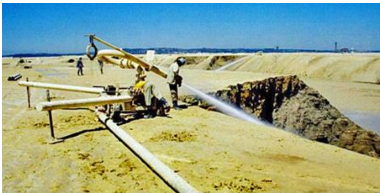
Figure 2 Hydraulic mining of gold tailings in Johannesburg prior to re-processing (source: Tailings.info 2015)
