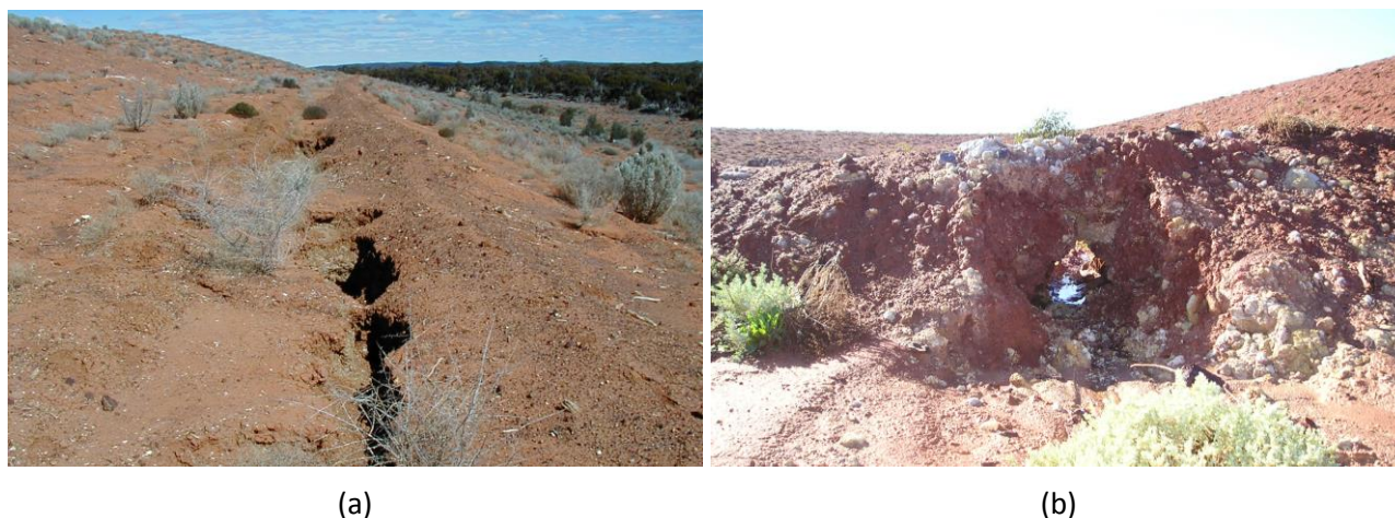
Figure 15 Contour drain in dispersive waste rock, showing: (a) tunnelling inlets along contour drain, and (b) major tunnel outlet, prior to collapse to form a gully
