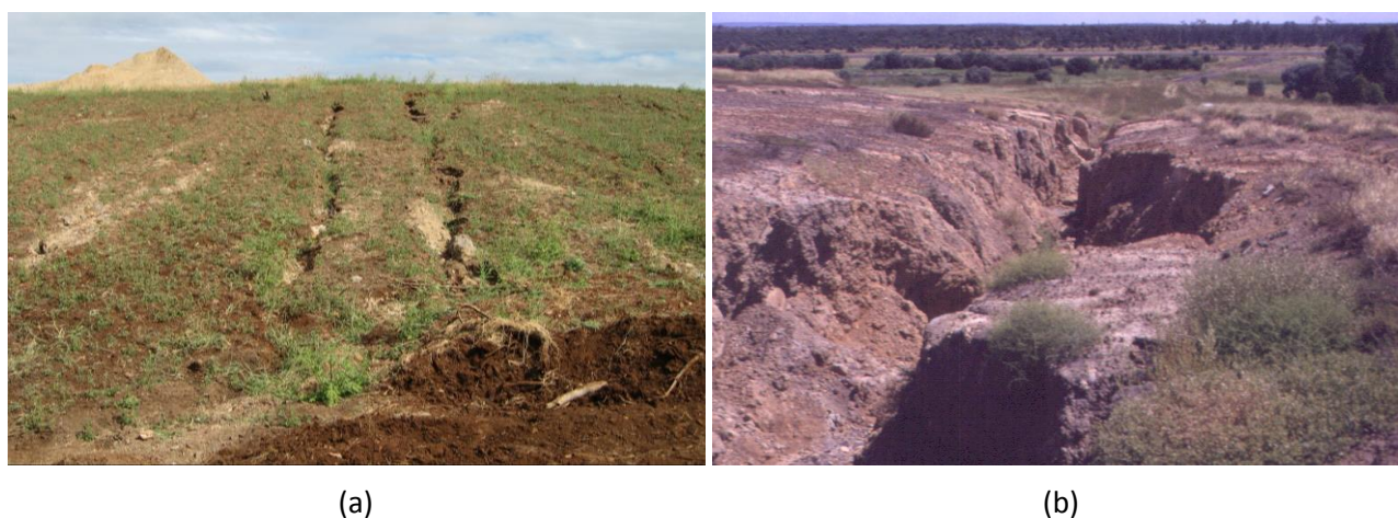
Figure 9 Flattened Bowen Basin spoil piles, showing: (a) rill erosion of grassed topsoil, and (b) failing downslope drain
