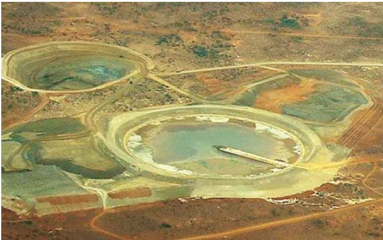
Figure 4 Aerial view of the IWL during construction
