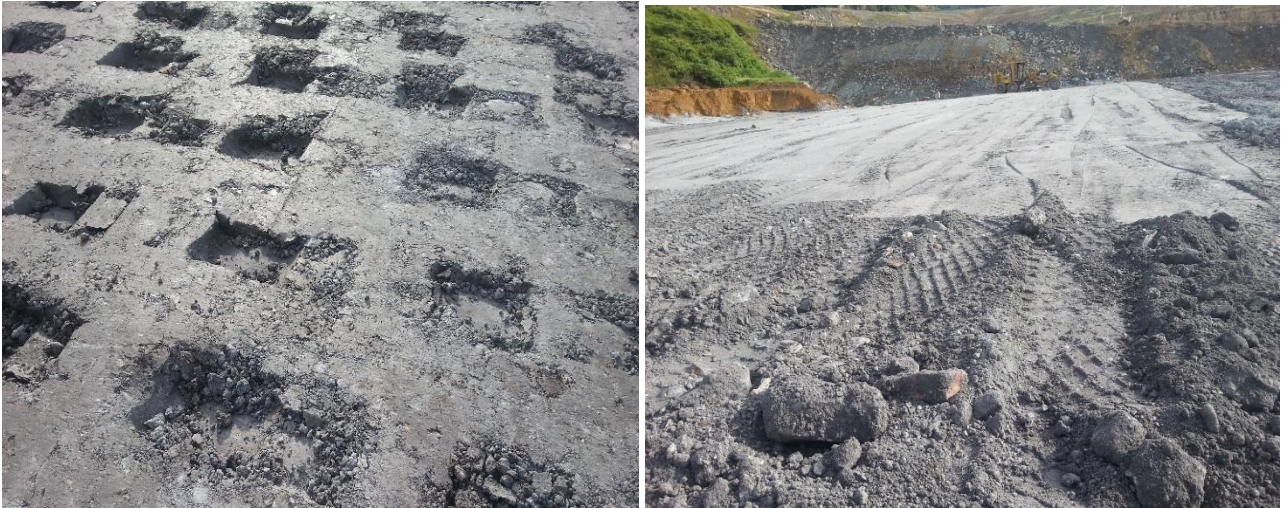
Figure 10 Site compaction on ROM material achieved using a roller. Note what appear to be large rock fragments are clumps of clay breccia which are readily broken down by compaction
