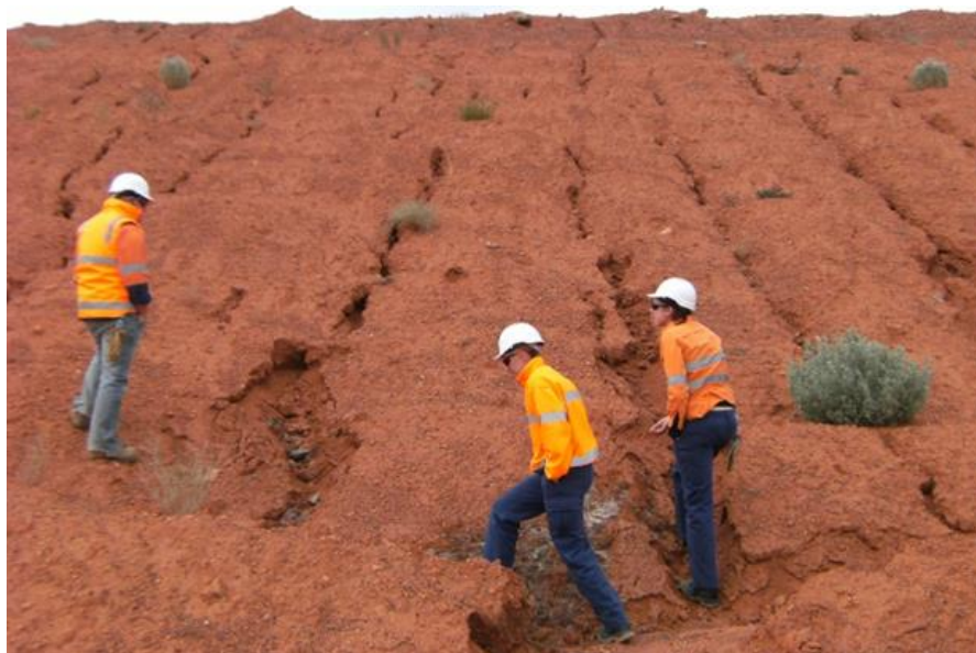
Figure 6 Over steep mine waste landform batters requiring repair
