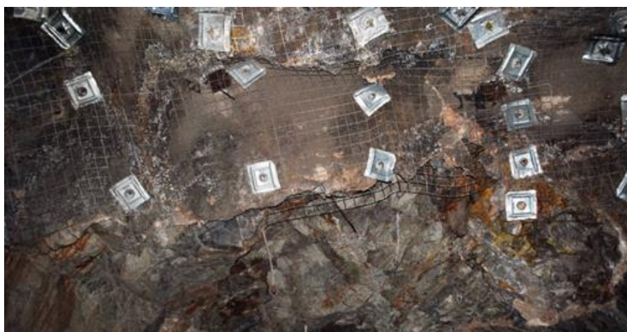
Figure 1 Damage in the backs of a development drive from a M_L2.9 seismic event at Mine A
