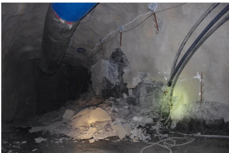
Figure 3 Ground failure in the main decline of Mine B triggered by a seismic event M_L 1.5
