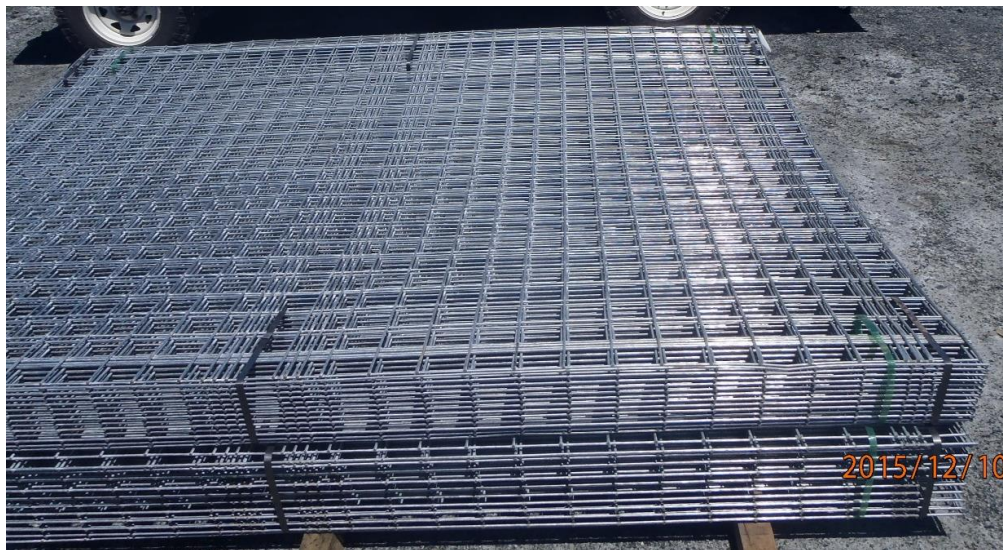
Figure 3 'Seismic mesh' delivered to site showing additional cross wires
