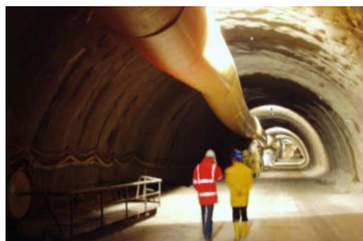
Figure 3 Smooth duct installed
