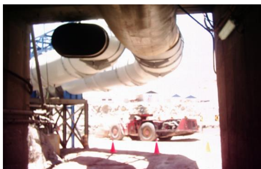
Figure 2 Oval duct installed
