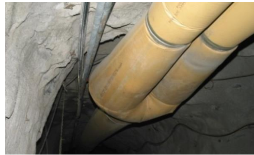
Figure 5 Smooth duct (duo) installed
