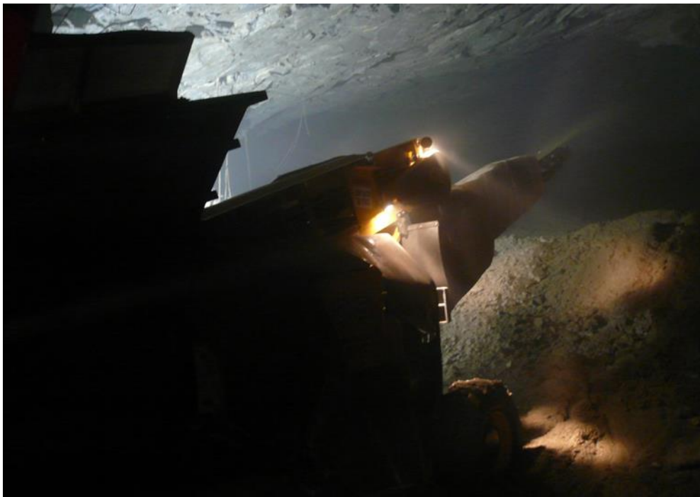
Figure 3 Filling voids underground
