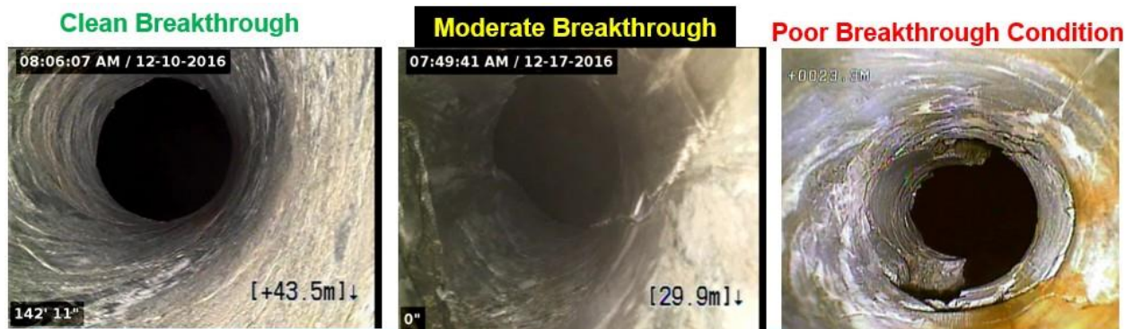
Figure 2 Borehole camera survey observations of breakthrough condition into underground voids
