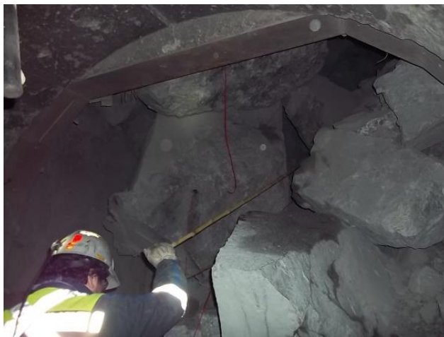
Figure 1 Current practice of a miner inserting explosives into low hang-up
