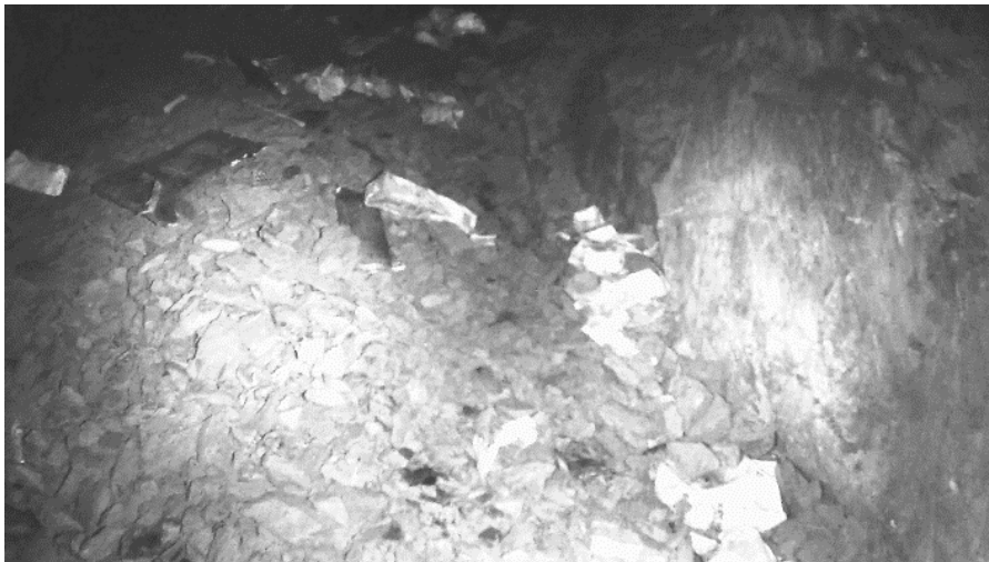
Figure 6 Rockfill and debris at base of stope (flights two and three)
