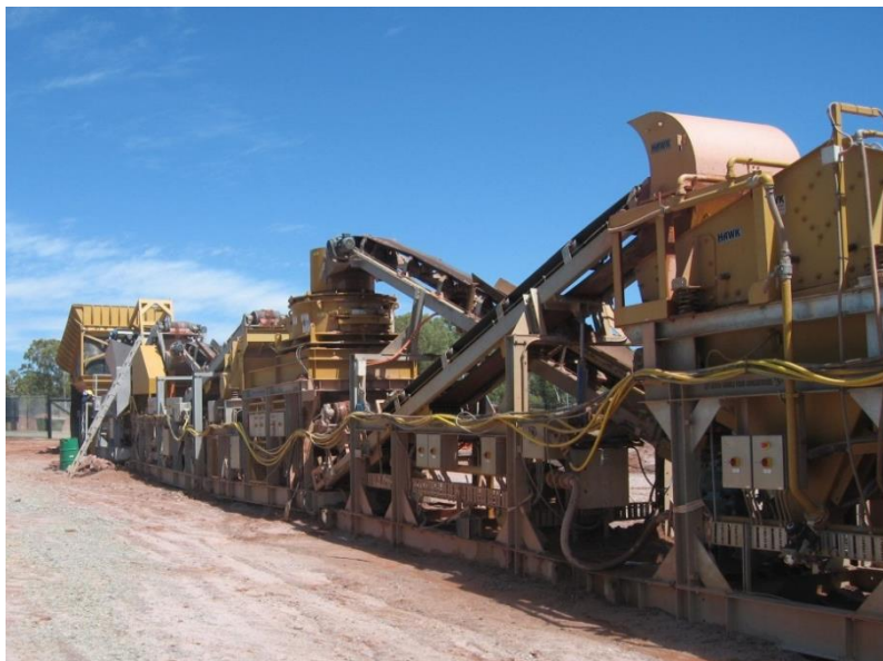
Figure 9 Python 200 installed and operating on a 1:50 slope
