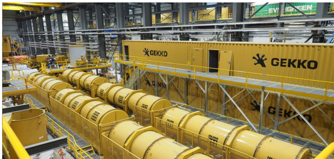
Figure 13 Hope Bay – modular Python plant and concentrate treatment plant (CTP)
