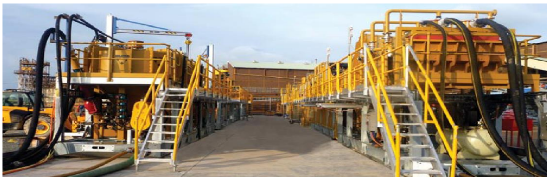
Figure 12 Python 500 installed and operating on a 1:50 slope
