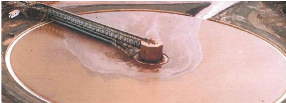
Figure 1 Un-collected fines short circuiting to the overflow
