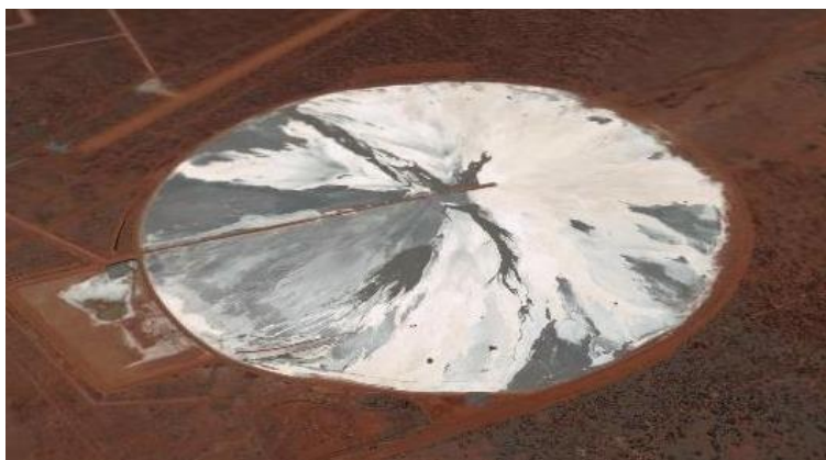
Figure 1 The Sunrise Dam CTD in Australia, operating since 2000 (Note the decant pond to the left)
