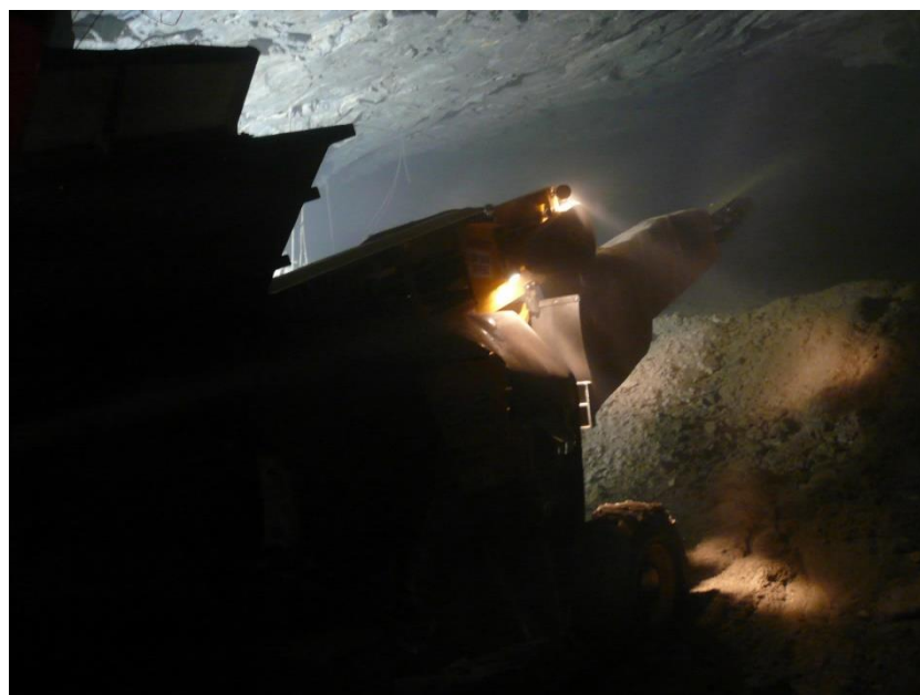
Figure 3 Filling voids underground
