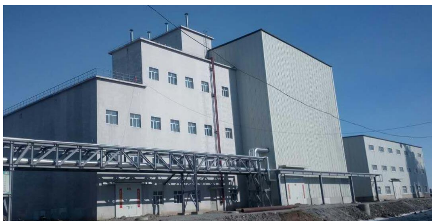
Figure 9 Outside view of the filling station and tailings conveying pump station
