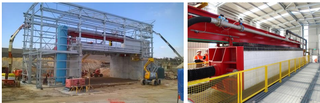
Figure 6 Overhead beam press being installed and commissioned in Victoria aggregates facility
