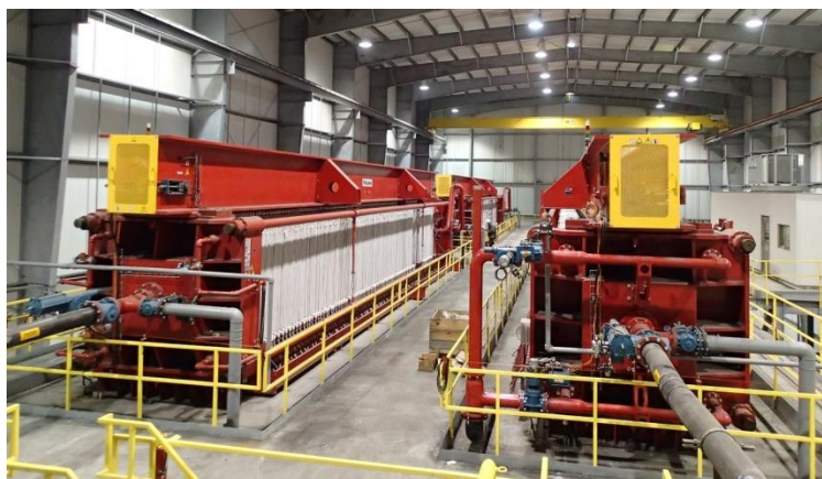
Figure 5 Inside the Indiana filtered coal refuse facility
