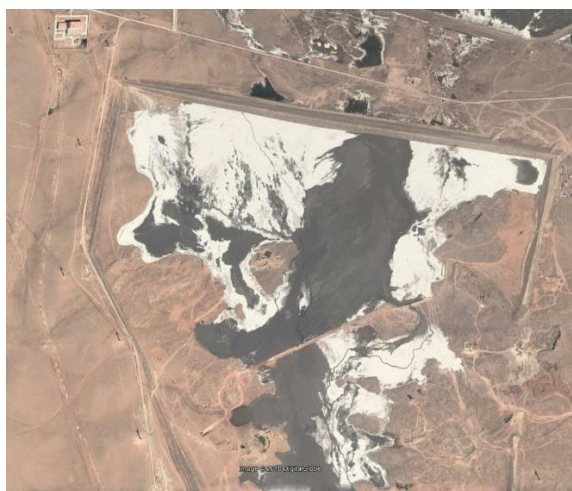
Figure 1 Baotou Steel surface stack layout showing the ~2 km down valley dyke
