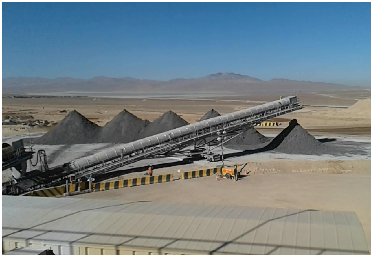
Figure 6 Stacks of dewatered tailings being created by the demonstration plant
