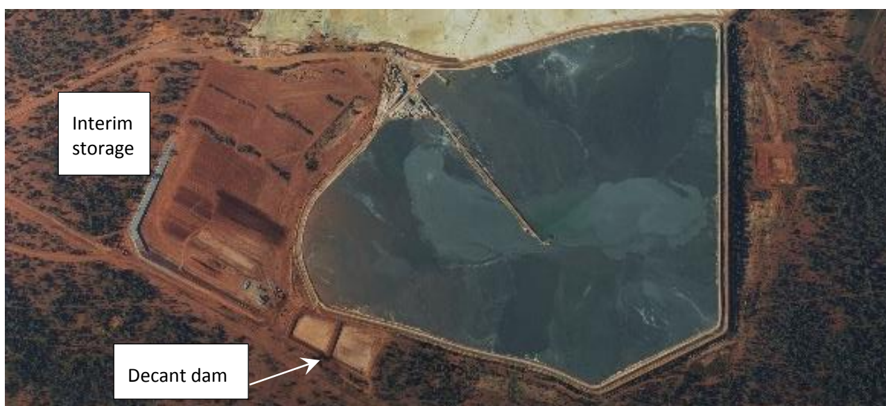
Figure 2 Aerial photograph of the South TSF during construction of the interim storage, September 2006
