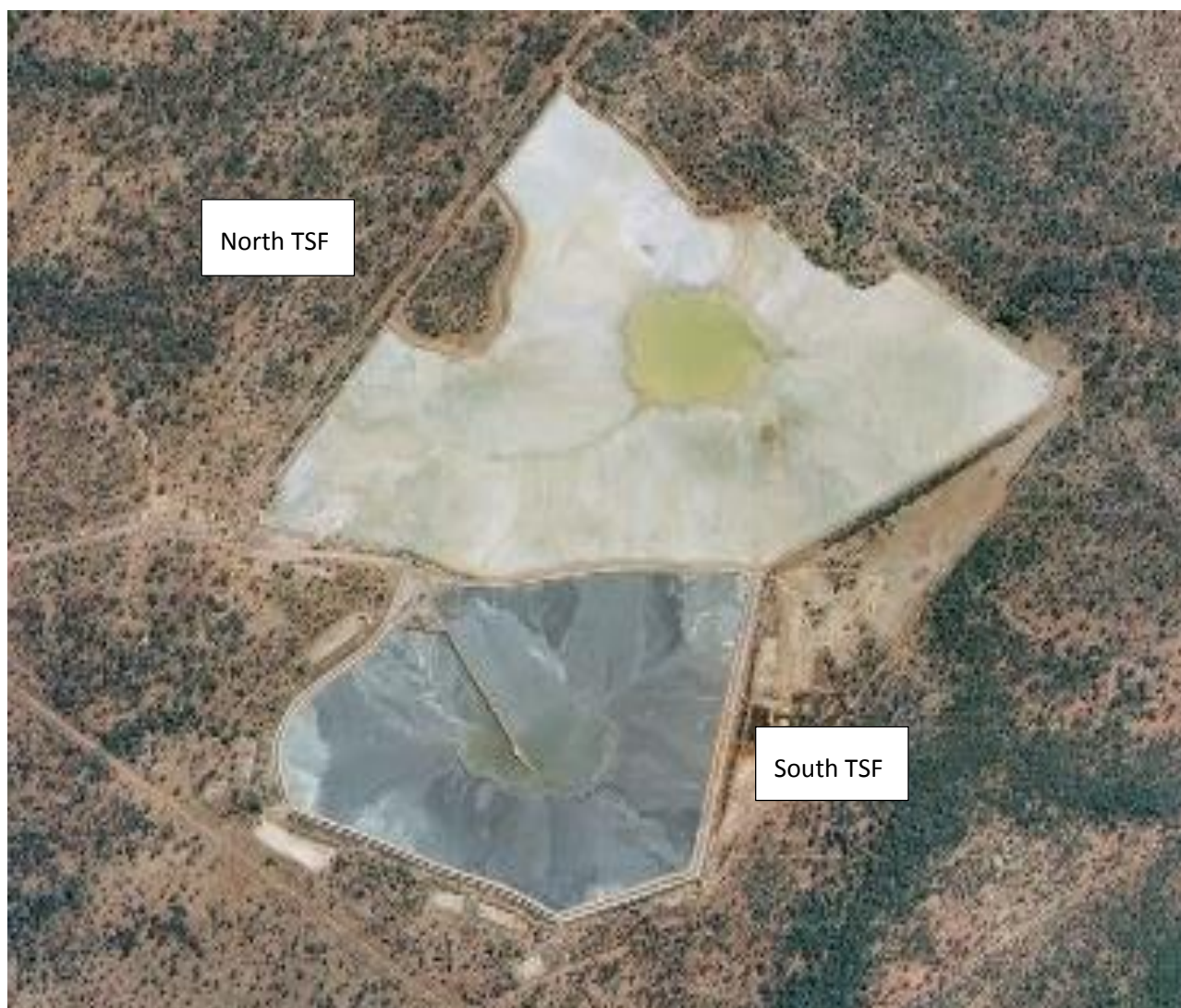
Figure 1 Aerial photograph of the site TSFs, dated August 2004
