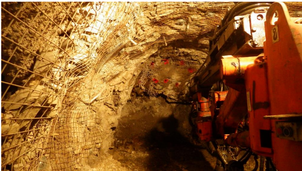
Figure 8 Excavation through the backfilled zone. A backfilled drawpoint is to the left. The lower portion of the backfill was excavated by LHD, prior to drilling and blasting the upper portion
