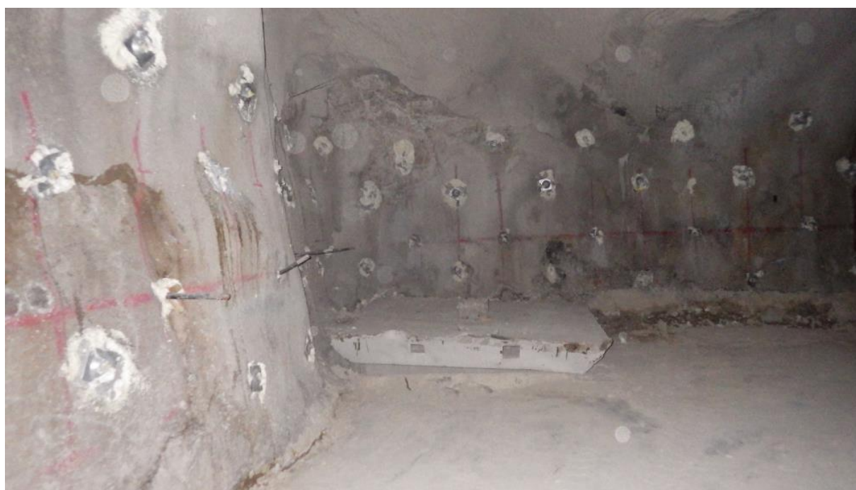
Figure 7 Friction bolts and hollow bar installed through the re-opened orepass for lower rib grouting
