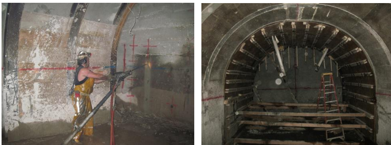
Figure 5 Re-mining through a collapsed extraction drift at Henderson in 2010. Cast concrete and steel arches were placed with each advance (from Carlson et al. 2012)
