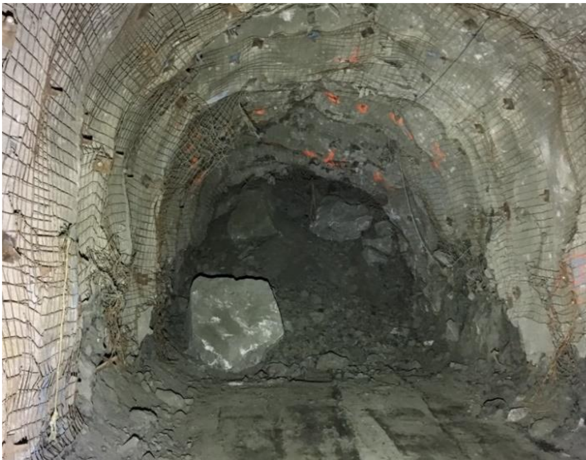
Figure 12 Granite wallrock oversize dilution in the A418 drawpoint
