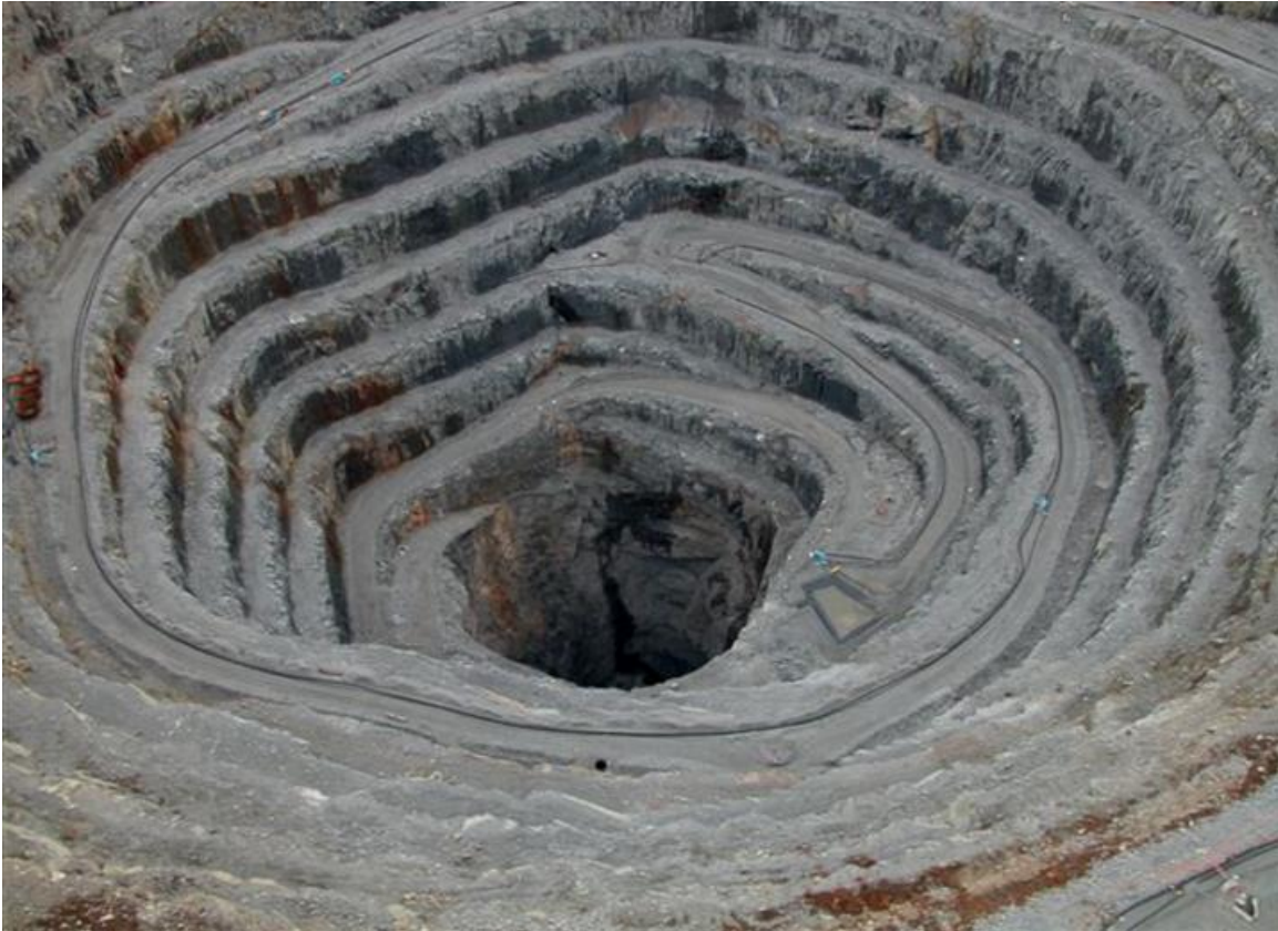
Figure 6 Empty SLR stope at the bottom of the Panda open pit
