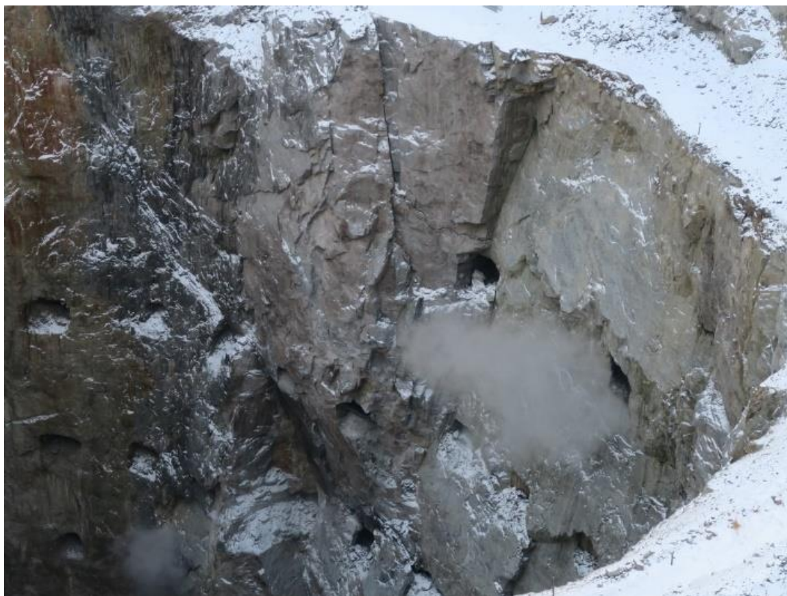
Figure 11 Wallrock failure at the A418 pipe at Diavik Diamond Mine
