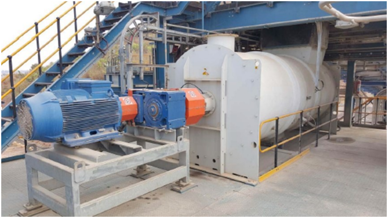
Figure 6 Paste mixer of thickened tailings for underground paste preparation
